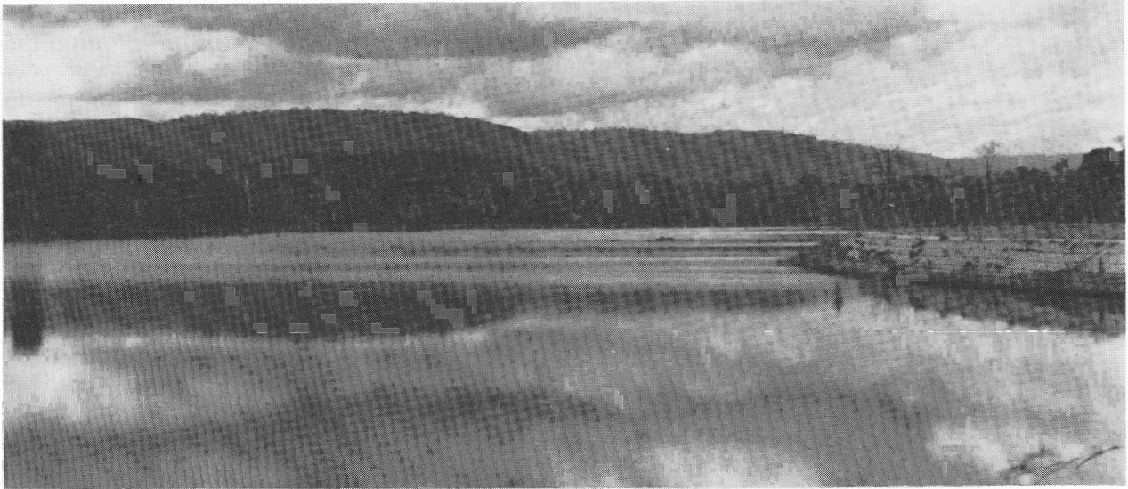
Figure 2. A settling pond (Barragem Esteril Norte) to trap sediment from mining operations at Serra dos Carajás, Pará, Brazil, February 1990.
