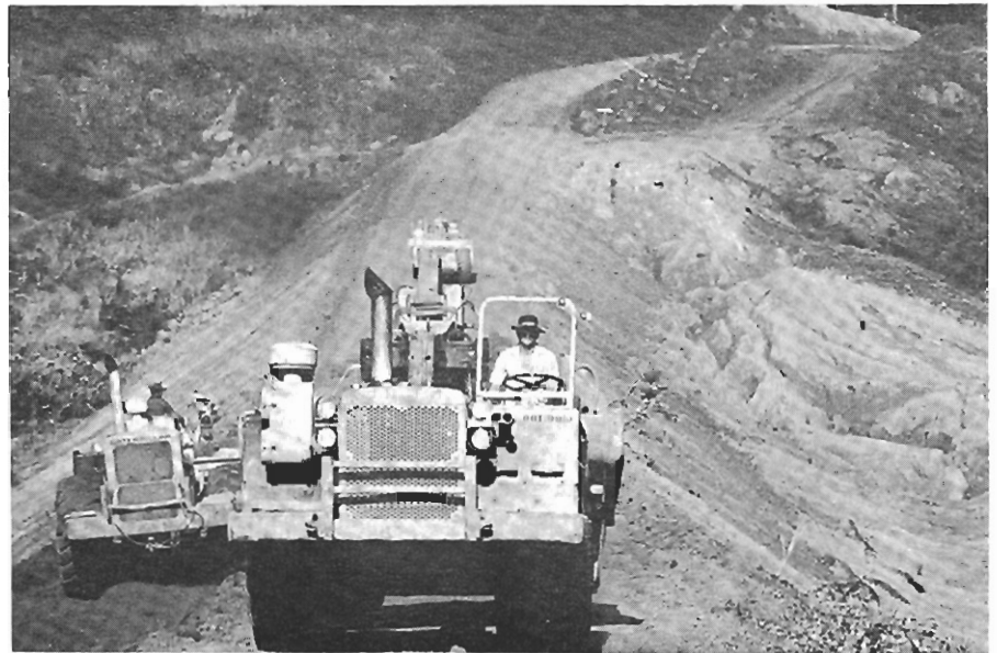
Fig. 2. Repairing the Transamazon Highway after the 1974 rainy season.
